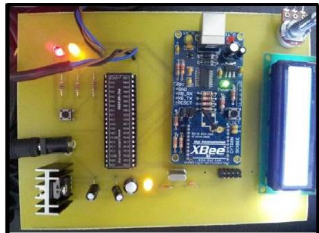
Fig 4: Circuitry Board of the Parking Lot Vacancy Monitoring Module
